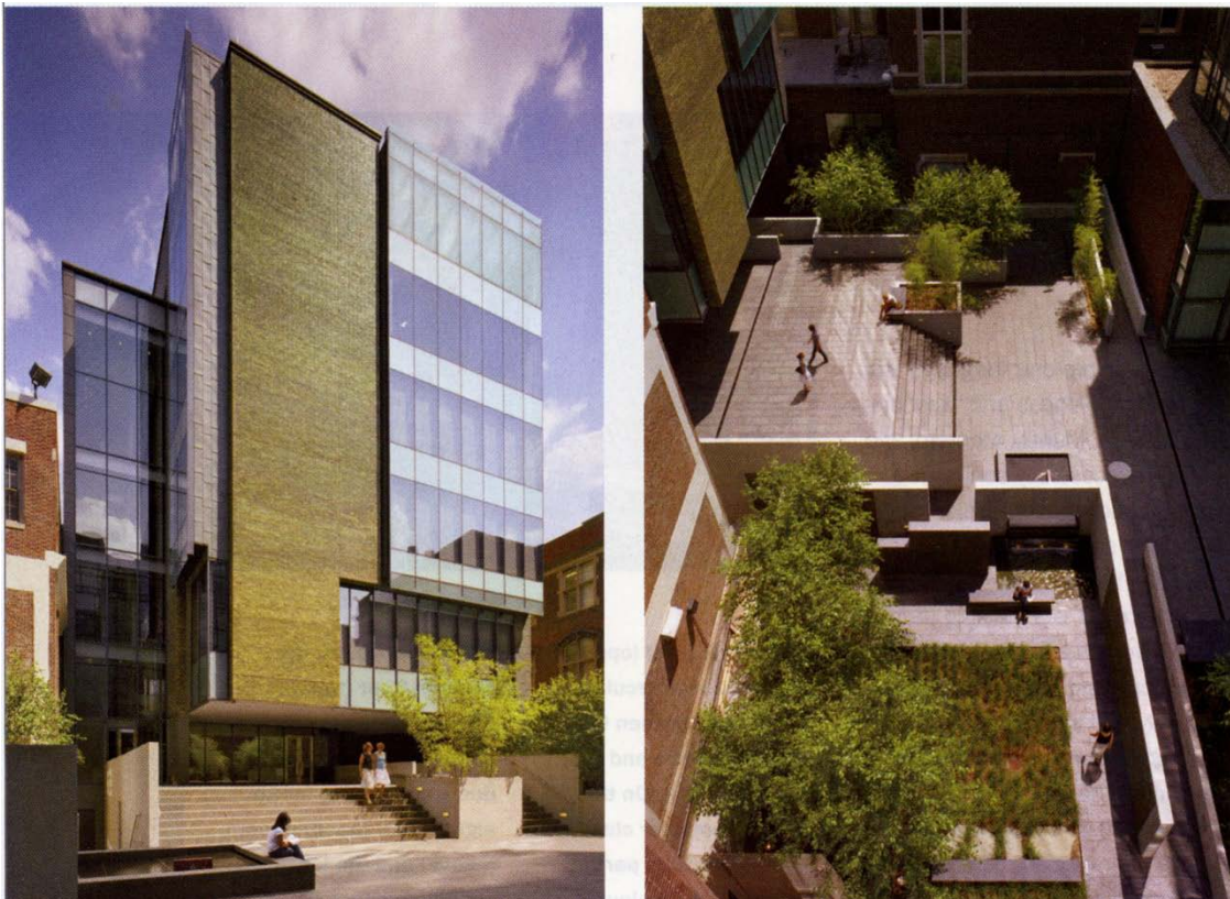
Skirkanich Hall, Tod Williams and Billie Tsien Architects, 2006. Photographs by Michael Moran for Architectural Record, 2007.
